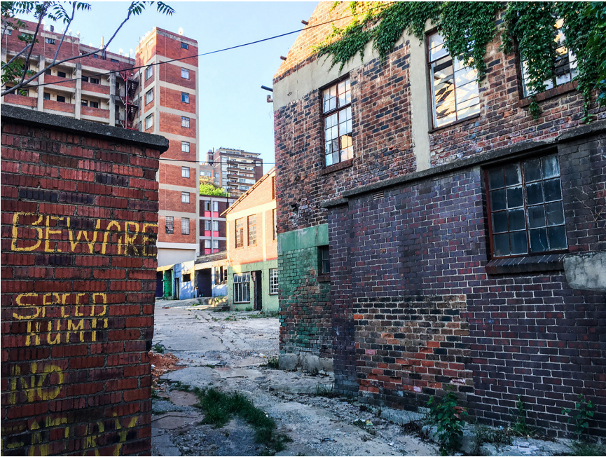
Figure 1. The now-empty carpet factory of 7 Saratoga Avenue, the center of the Blue Moonlight case. Photo by Matthew Wilhelm-Solomon, 2017.
