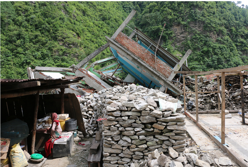
Figure 4. Waiting to rebuild. Photo by Aidan Seale-Feldman.
