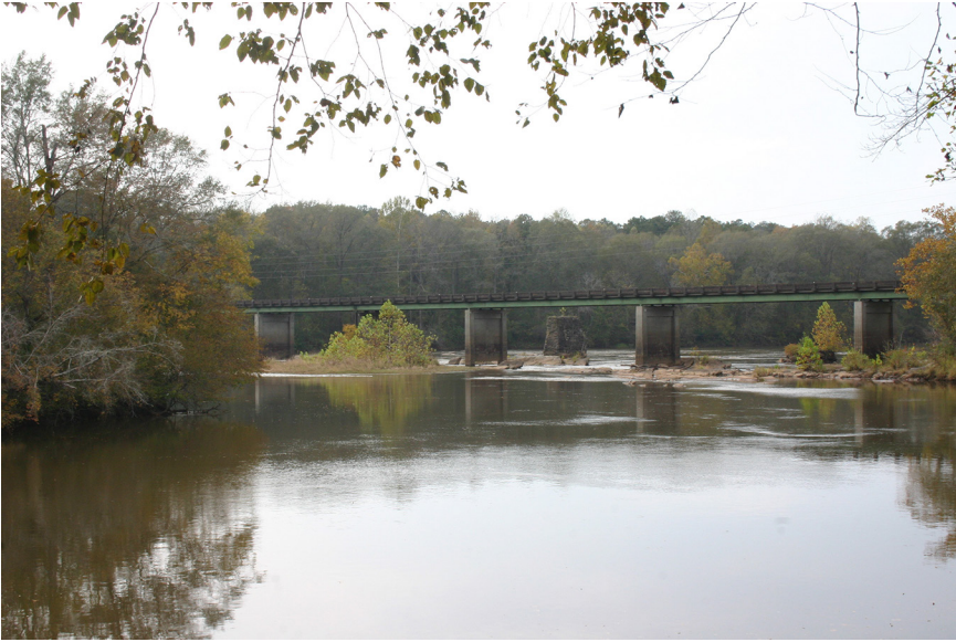
Figure 7. An old bridge falls into the Tallapoosa River at Horseshoe Bend. A new bridge has been constructed in front of it. Photo by Leigh Bloch.
