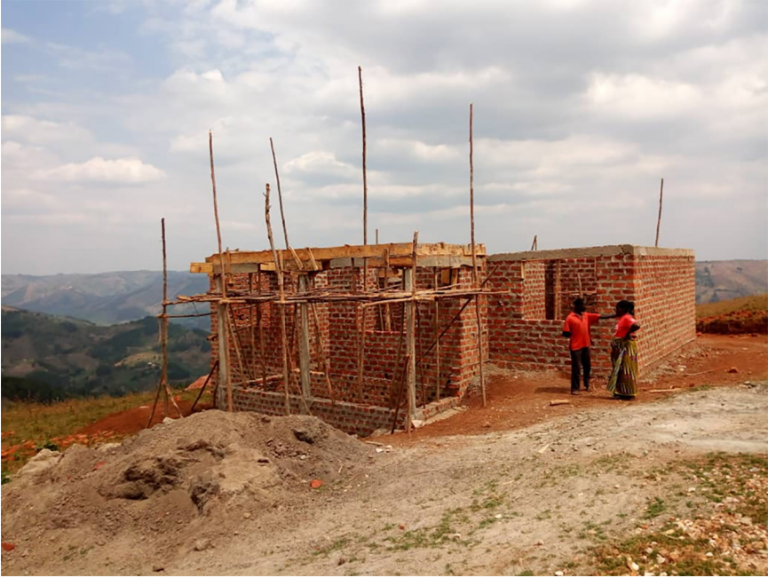
Figure 1. A small, half-built, brick house on the outskirts of Mbarara. This modest construction project was already two years in the making when this photo was taken. Photo by Twesigye Pius.
