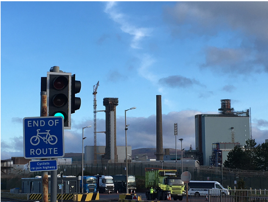
Figure 5. Legacy facilities on Sellafield site in the process of being decommissioned, close to the main gate where trucks are inspected before they are allowed to enter the site, 2019. On the left (with the crane perched above it) is the Pile One chimney where the 1957 Windscale fire occurred. Photo by Petra Tjitske Kalshoven.
