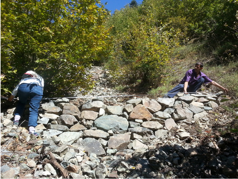
Figure 6. A forester and a villager are measuring the erosion control walls built in Gudashev within the scope of the watershed rehabilitation project. Photo by Ekin Kurtiç.
