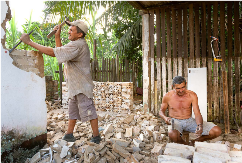
Figure 4. Unbricking an entire house on Perimetral Avenue, Altamira, Pará, 2015. Photo by Carlos Fausto.
