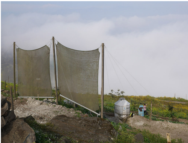
Figure 1. Worn-out fog catchers above Villa Fátima, September 2018. Photo by Chakad Ojani.
