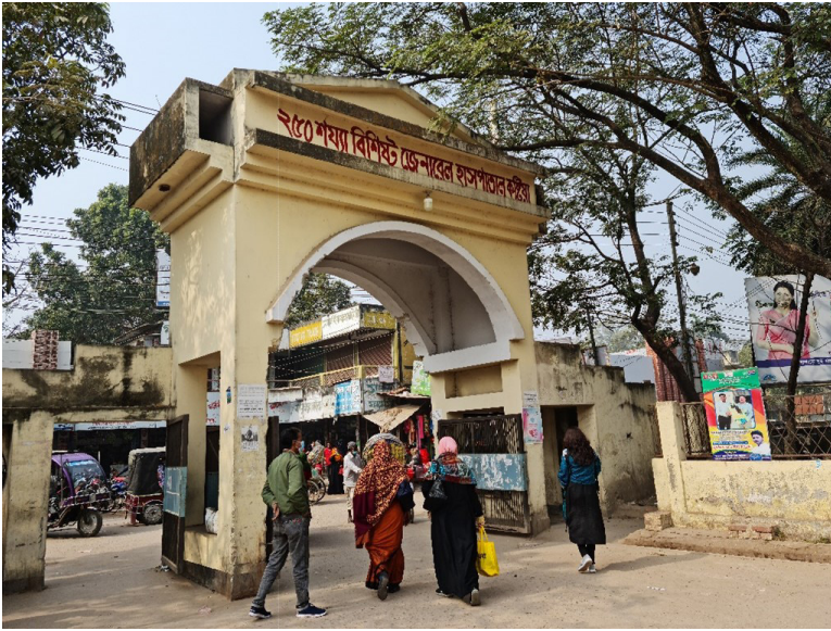
Figure 1. Entry gate of the Kushtia district hospital. Photo by Janet Perkins.
