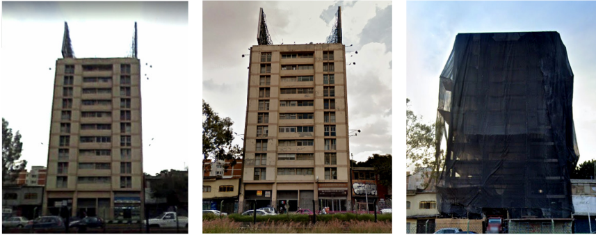
Figure 6 (left). Calzada Tlalpan 1178, December 2008. Figure 7 (middle). Calzada Tlalpan 1178, September 2017. Figure 8 (right). Calzada Tlalpan 1178, November 2021. Photos from Google Maps.
