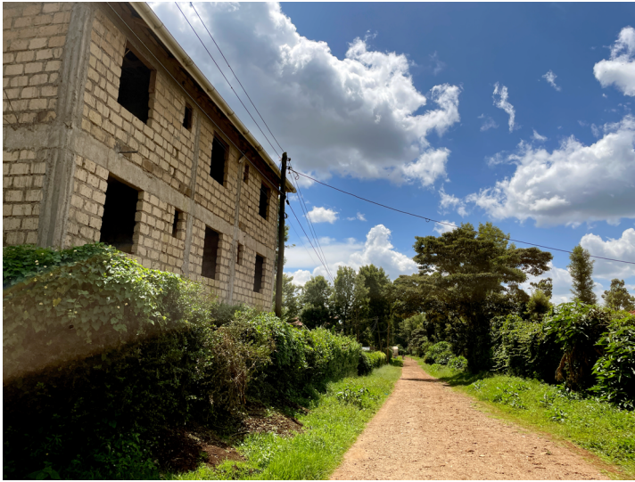
Figure 3. Rental ‘plots’ under construction in Ituura. Photo by Peter Lockwood.
