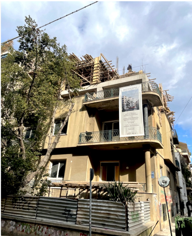
Figure 5. Construction of Peloria 2, May 2022.
